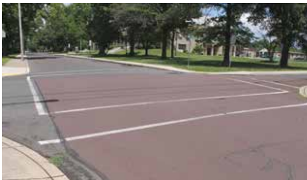
Standard crosswalk markings are less visible to drivers, but are preferable to having no painted crosswalks at all.
