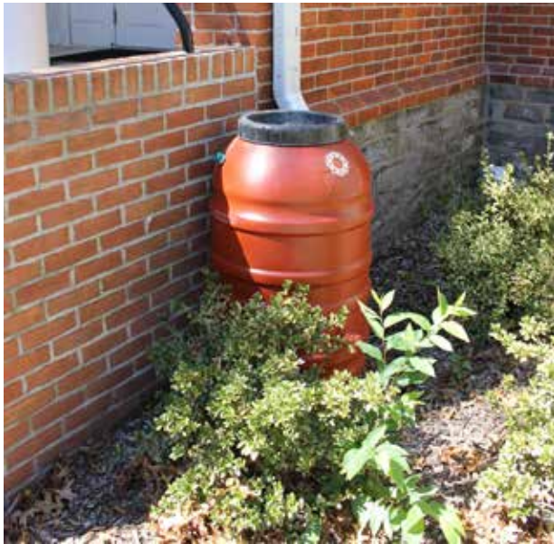
Borough Hall offers this style of rain barrel to residents. Captured water can be used to water lawns and gardens.
