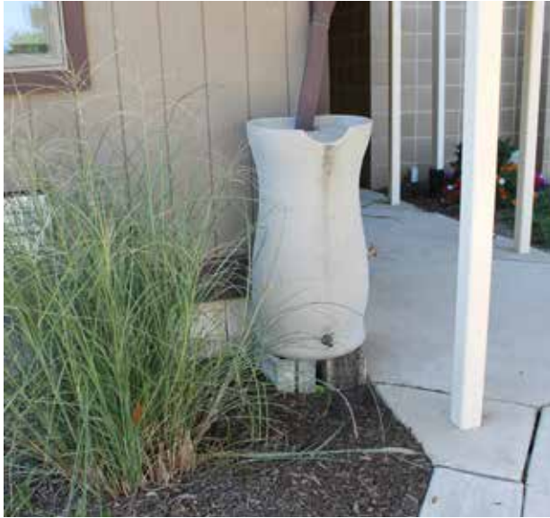
Rain barrels, such as this one at North Wales Elementary School, can be used to capture stormwater runoff.
