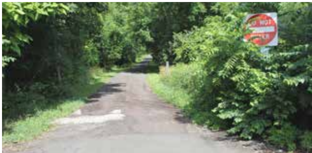
The entrance to the Parkside Place Park trail connection is poorly marked and overgrown with vegetation.
