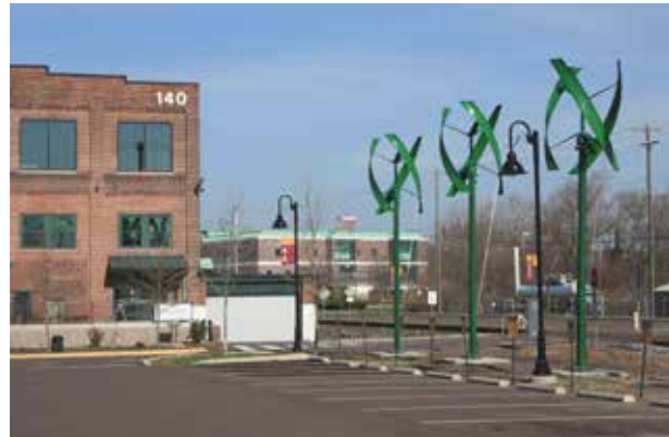
Small-scale vertical axis wind turbines at the Montgomery County Community College campus in Pottstown Borough are an example of wind energy infrastructure in an urban context.
