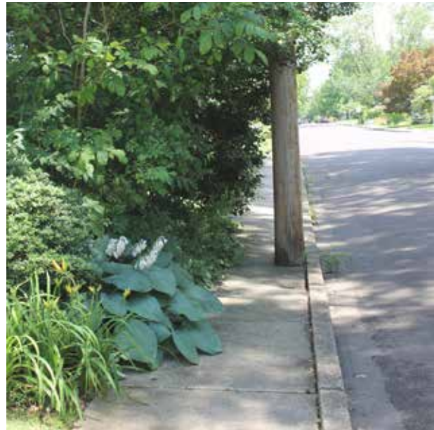
Overgrown vegetation and utility poles limit sidewalk widths, making it challenging for stroller and ADA access and cause pedestrians to move into the roadway to avoid obstructions.
