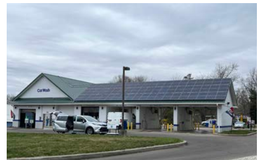
Solar Panels on Captain Carwash, Worcester Township
