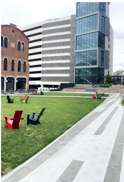
SORA West, the county's first C-PACE approved project, Conshohocken Borough
