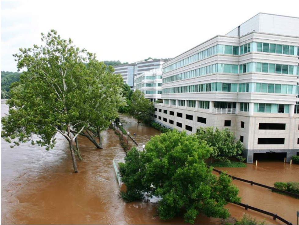
Flooding Tower Bridge II, West Conshohocken Borough
