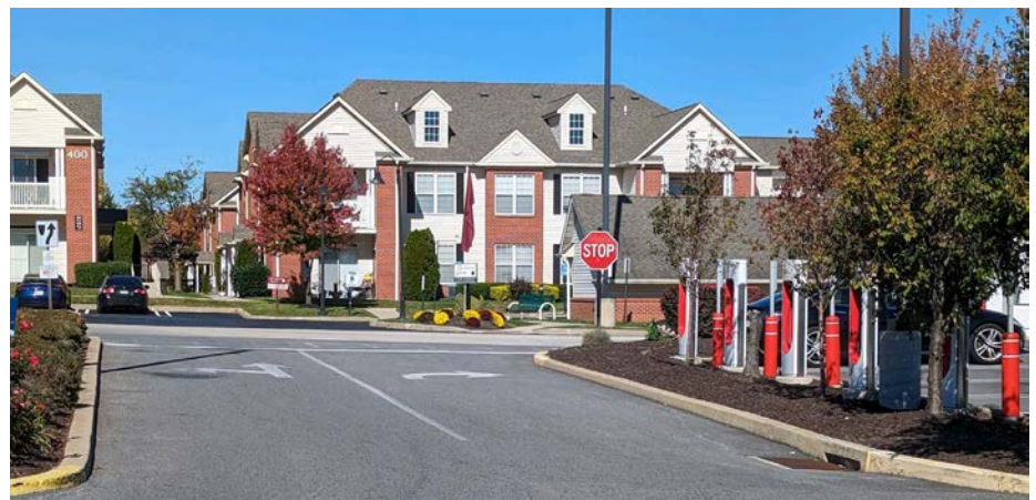
Multifamily housing and commercial areas provide locations for EV charging stations, Upper Merion Township
